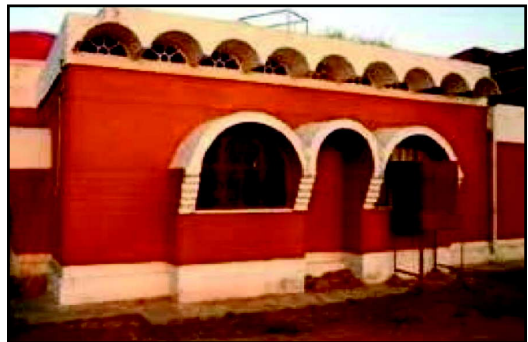
Figure A3.19. Ferro-Cement Roofing
