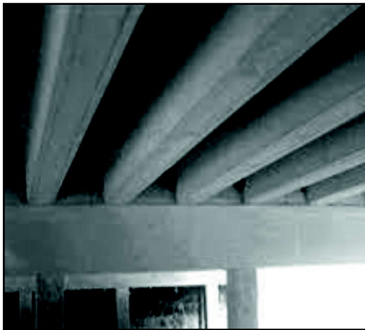
Figure A3.18. RCC channel units
