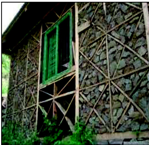
Figure A3.13. Dhajji-diwari walling System Image
