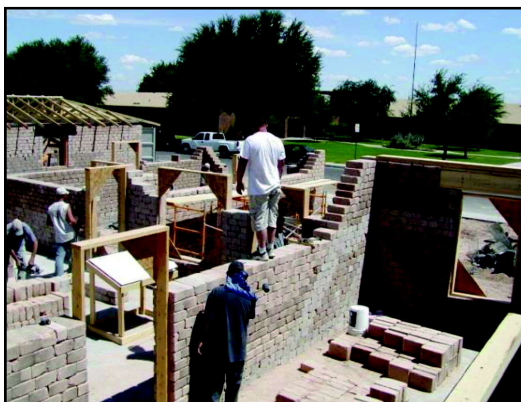
Figure A3.9. Compressed earth block masonry system Image
