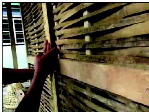
Figure A3.11. Bamboo strip walling
