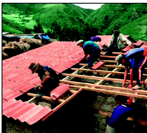
Figure A3.14. Micro-concrete tiled roofing
