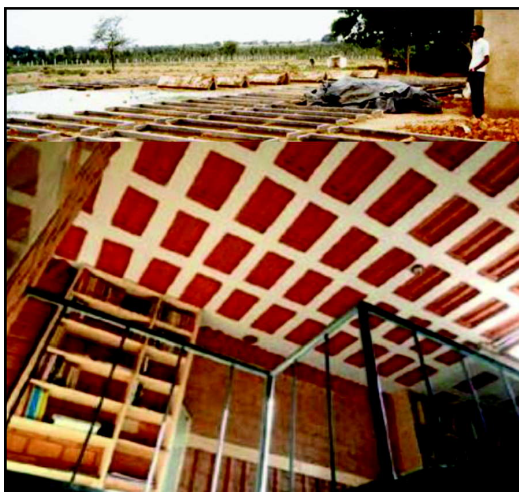
Figure A3.17. 'L' panel (above) & Filler slab roofing
